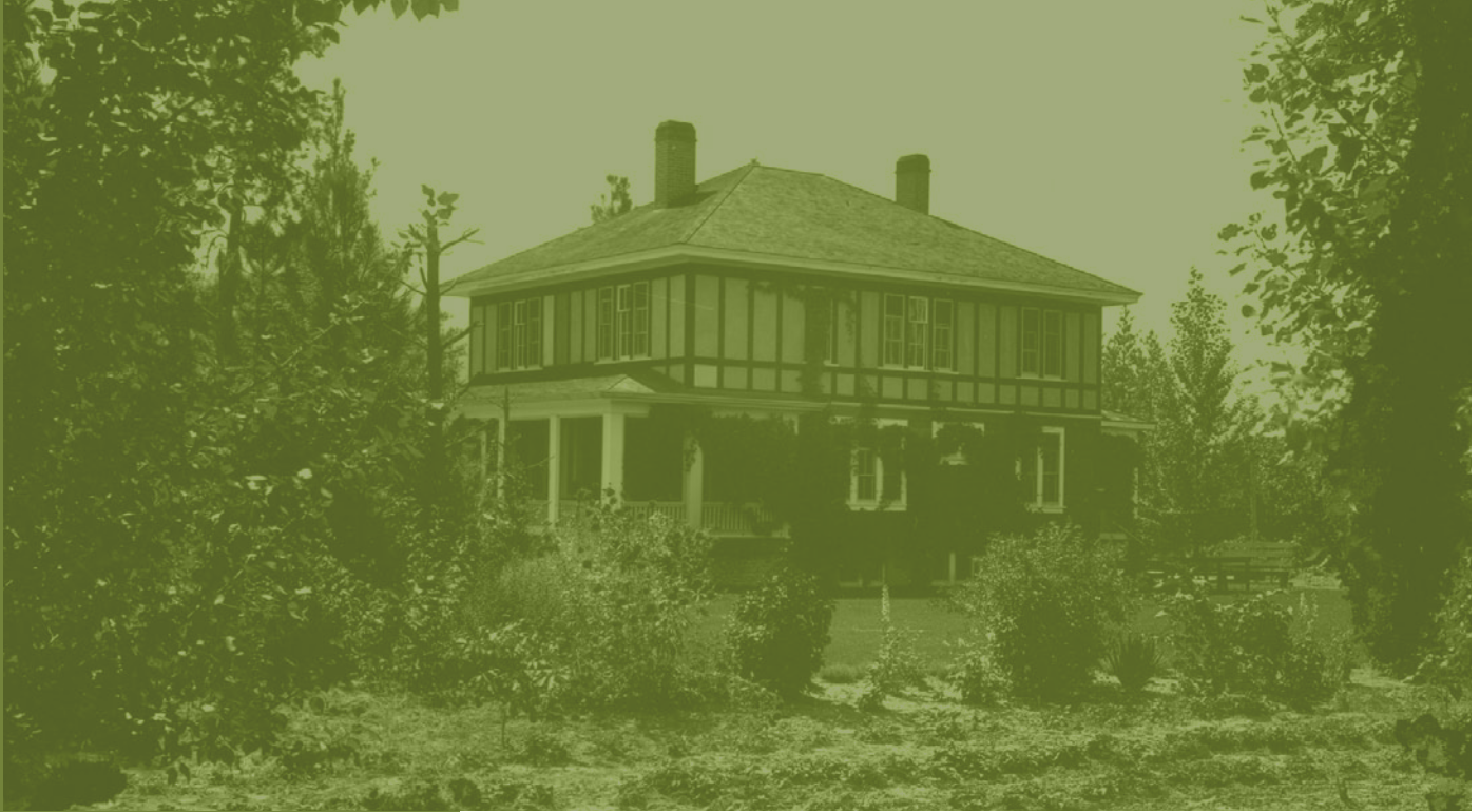
Belgo House, 1590-1640 Belgo Road
