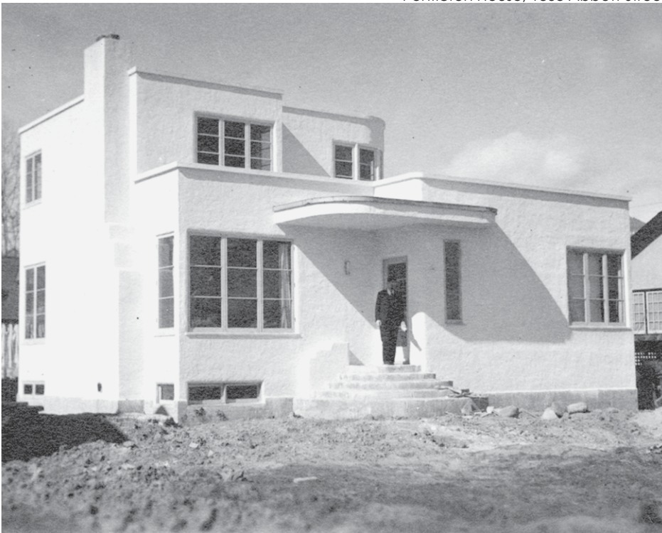
Penticton House, 1858 Abbott Street
